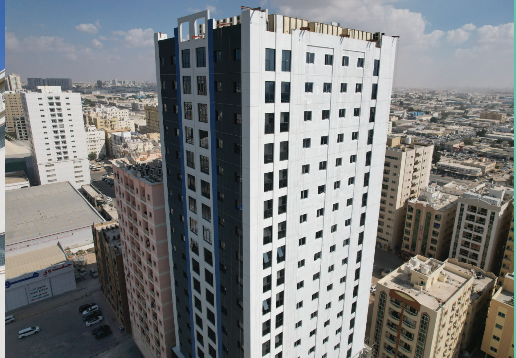
G+5P+16 Building at Industrial Area 2, Ajman
